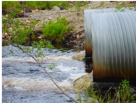
Above: Current culverts are perched and undersized, presenting a barrier to salmon moving upstream to spawn.
