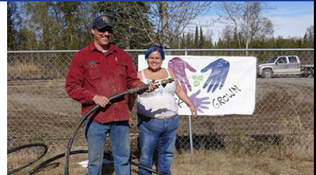
Above: Sam Bartels with new water line.
